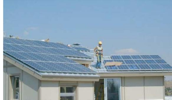
The PV panels are mounted on rails, which in turn are mounted directly to the metal ribs of the standing seam roofing using S-5 clamps. This is a unique mounting system that eliminates any penetrations through the weather sealing of the roof and therefore preserves the integrity of the building envelope.
